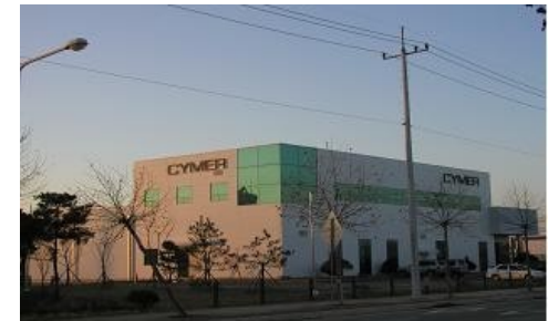
Demonstration Facility and Integration Center Pyongtaek, Korea
